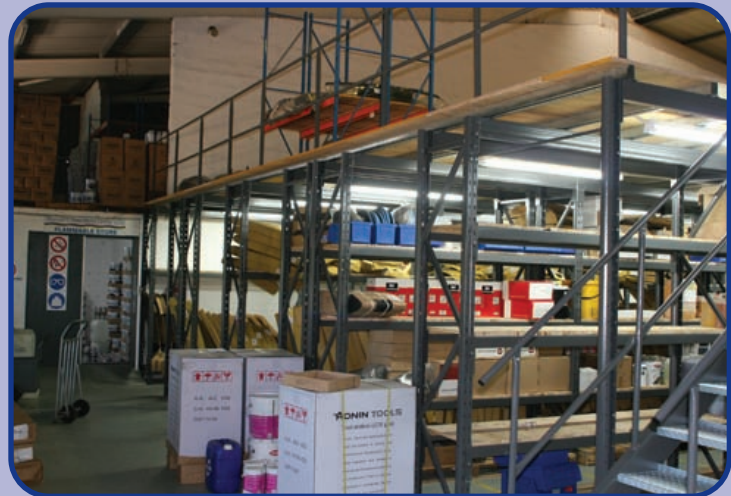
RACK SUPPORTED MEZZANINE FLOOR
