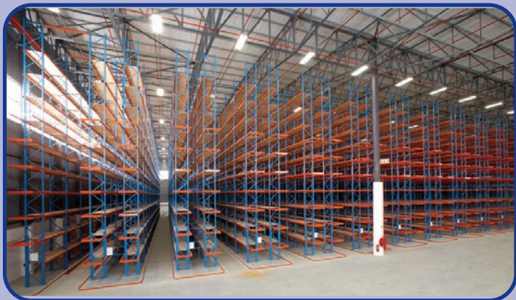
NARROW AISLE RACKING
